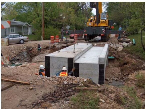
Construction of Elm Street Box Culvert Replacement, March 18, 2005
